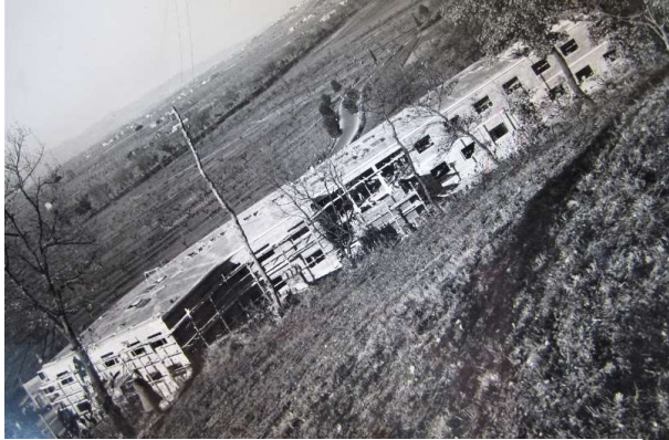
The construction of the new factory at the new location.
