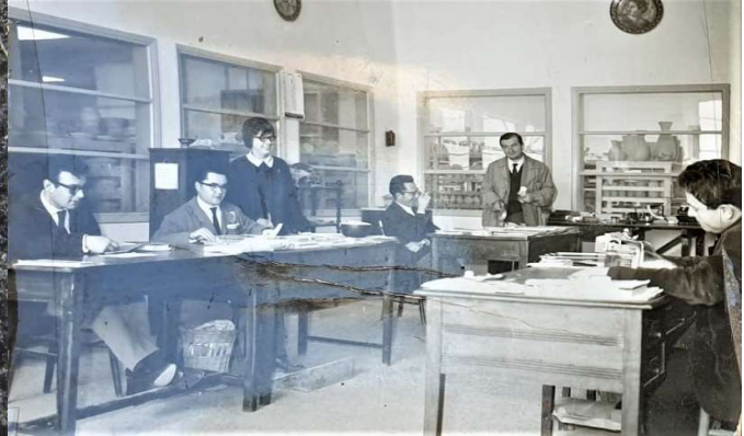
Francesco Baiano in the Offices of the factory.
