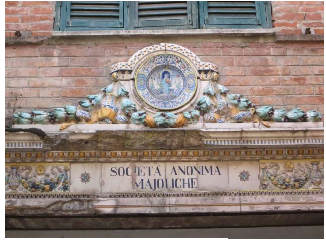
Main entrance to the factory
